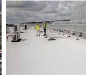
Exposed Roofs 外露屋頂
