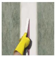
Apply the Combiflex SG tape within the open time of the adhesive. Press the tape firmly, without trapping air, into the adhesive using a suitable roller. The adhesive should be squeezed out on both sides of the tape by  $\sim 5$  mm.
