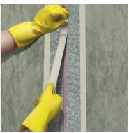
Apply the mixed Sikadur<sup>®</sup> adhesive on both sides of the joint / crack onto the prepared substrate, using a suitable brush, trowel or spatula.. If the concrete substrate is damp, force the adhesive firmly into the substrate. The layer thickness of adhesive should be 1 - 2 mm and the width on each side of the joint / crack at least 40 mm.
