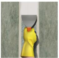
Before placing the Combiflex tape remove the masking tape on top of the central expansion joint / crack area.
