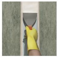
Remove the red middle strip and the masking tape on both sides to ensure a neat and precise detail.
