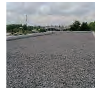
Gravel Ballasted Roofs 壓層礫石屋頂
