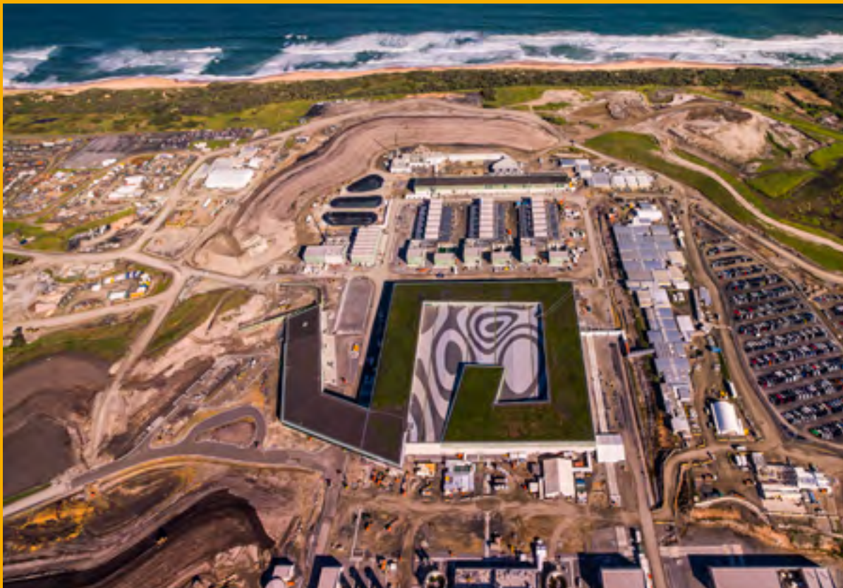
The Victorian Desalination Plant, Wonthaggi, Australia
