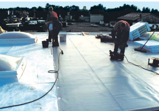
Recovering of waterproofing membrane
