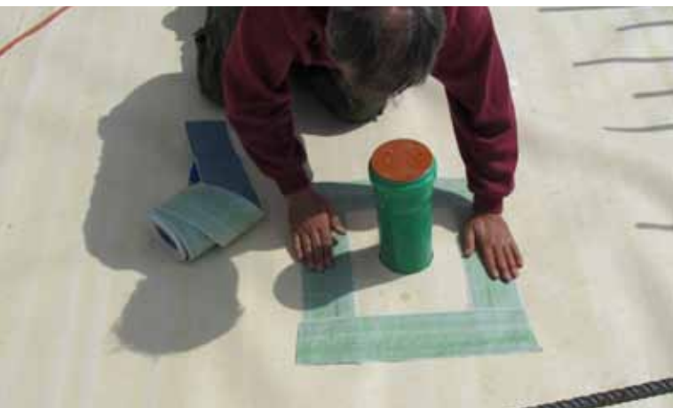
Internal jointing detail with SikaProof® Tape -150 .
