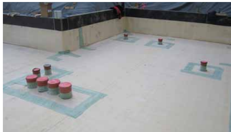
Finished internal jointing detail
