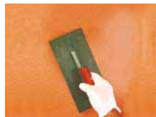
Sealing of a broadcast layer with a straight trowel or "squeegee" blade.
