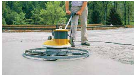
Power float with a variable speed control for trowel finishing of concrete and resin floors.
