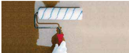
Primer application with medium pile roller.
